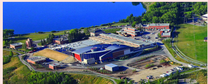
The Glenmore Water Treatment plant treats drinking water for people living in the south part of Calgary. Where does drinking water come from in your community, and where and how is it treated?
