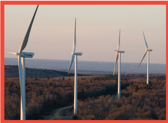
Wind turbines. Source: TransAlta Corp ( www.transalta.com ).
