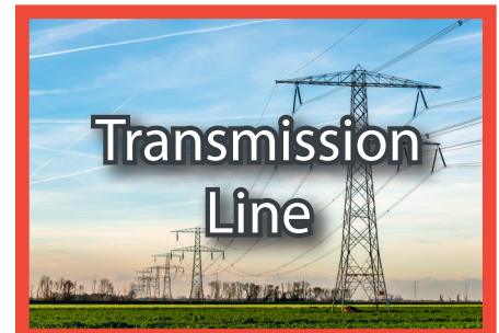
A transmission line carries electricity
