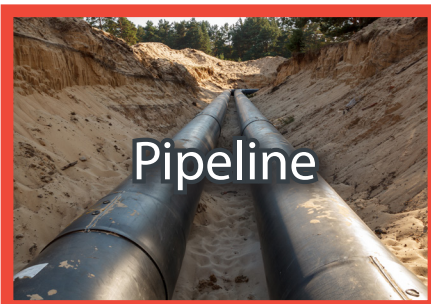
A pipeline carries oil or natural gas.
