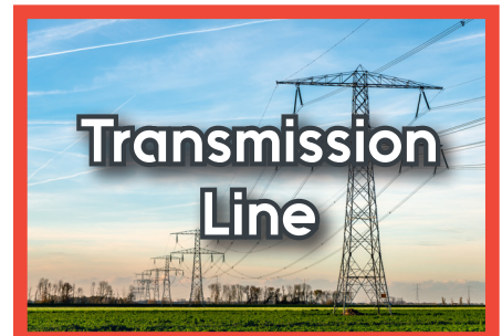
A transmission line carries electricity
